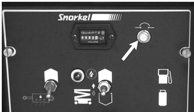
Figure 5.4 - Main Circuit Breaker
